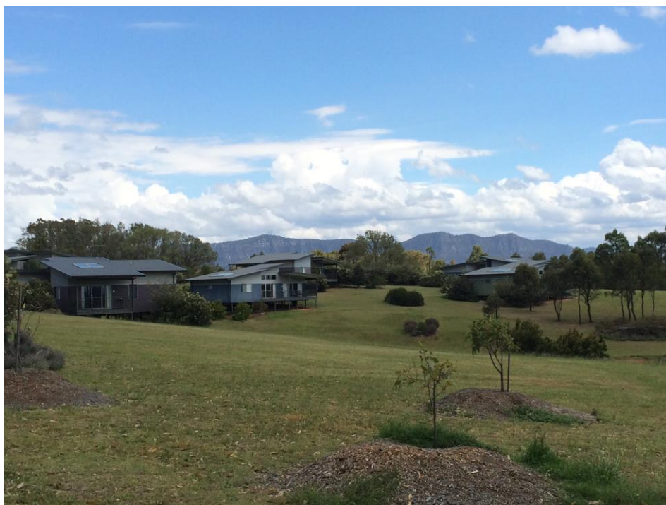
Figure 10 – Adjacent tourist accommodation, Old North Road Source: JBA
